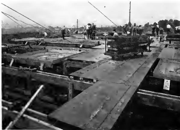
FIG. 5. PLACING THE STEEL PANELS
